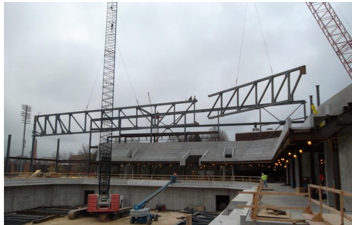
Figure 1 – First Truss Erected, 3/1/12, Courtesy of Gilbane
