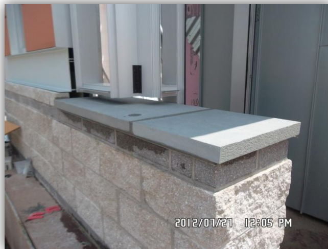
Exterior Masonry on Mock-up - Taken by Derek Stoecklein
