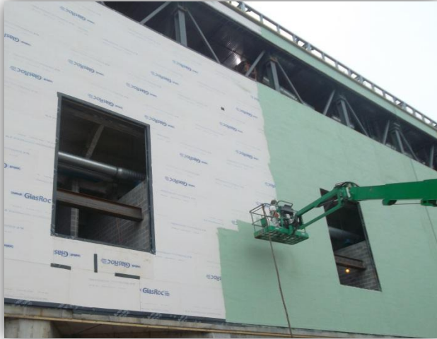
South Vapor Barrier - Taken by Derek Stoecklein
