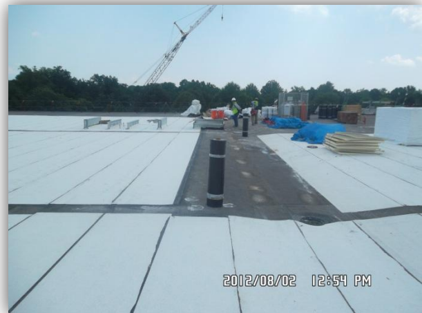
Roof base sheet - Taken by Derek Stoecklein
